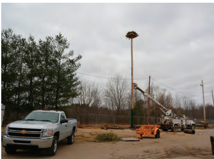
Installing the new nest platform before the Ospreys returned, 3-6-18.
